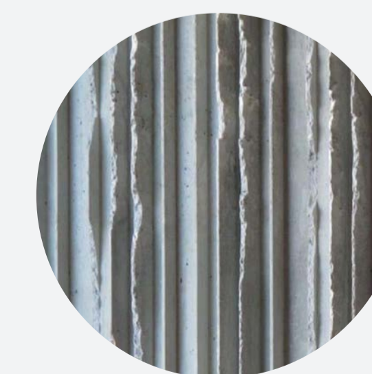
EXPRESSED FORMWORK UPPER FLOORS
