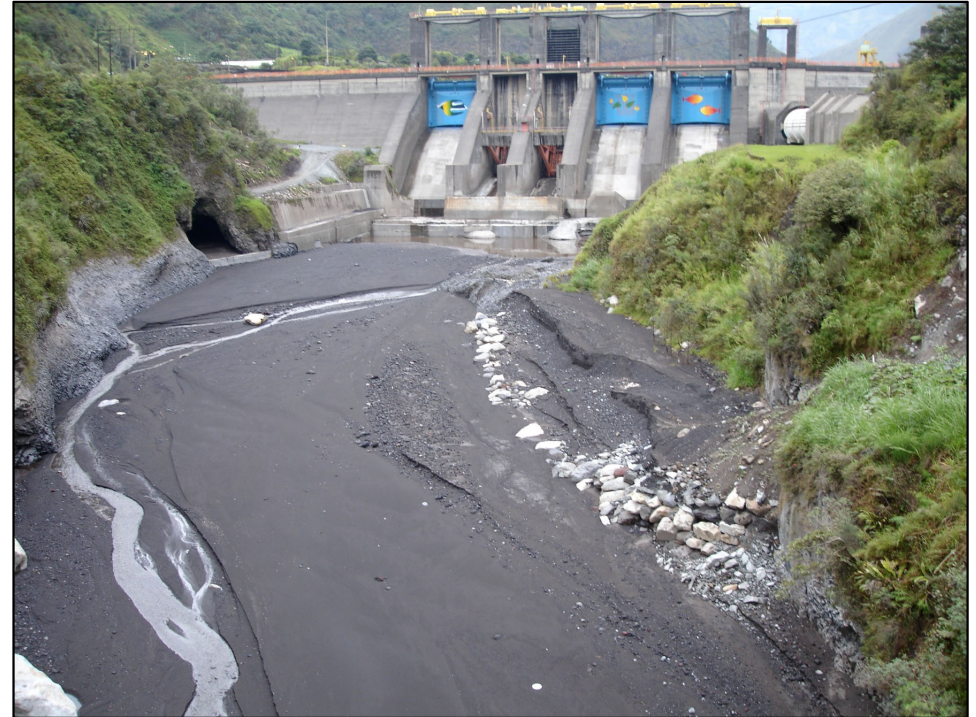
HidroAgoyan Dam, Pastaza River, Ecuador
