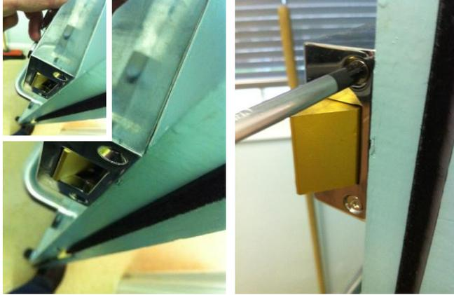
Once you have aligned the tail with the slot carefully slot the lock assembly back onto the bracket (see pictures). Replace the retaining screws and test that the latch works.
