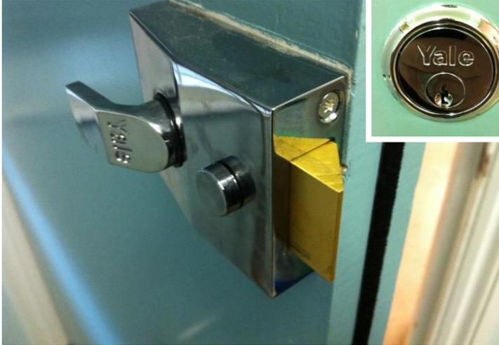
A night latch like the type pictured is a very common surface mounted lock (usually used in conjunction with a mortice or deadlock in a domestic setting).
