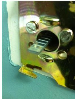
Use the key from the outside of the door to adjust the tail to a horizontal position (see pictures top)
