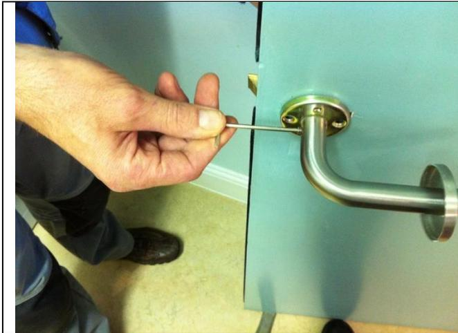
Next remove the Allen key (hexagonal key) grommet from the handle and set to one side (you may not need to do this to release the handle assembly).
