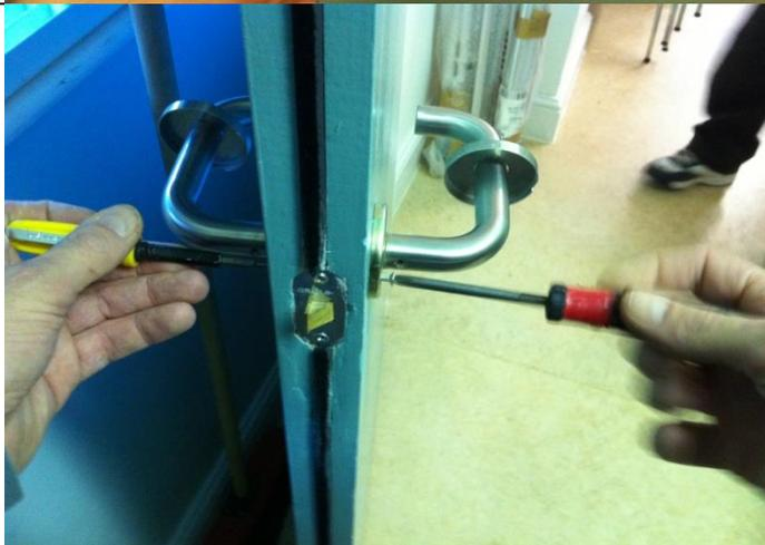
When removing the handle you find that the screws sometimes spin – if this happens remove the plate cover from the other side of the door (same method as the first step on this page).
