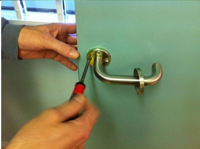
Once the surround has been removed remove the two screws that hold the handle on.
