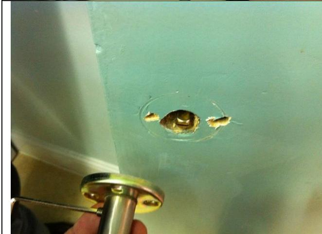
Remove the handle assembly from the door.
