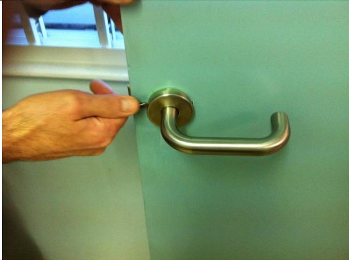
Remove the handle plate cover using a screwdriver as a lever; there is a small cut-out in the cover for this purpose.
