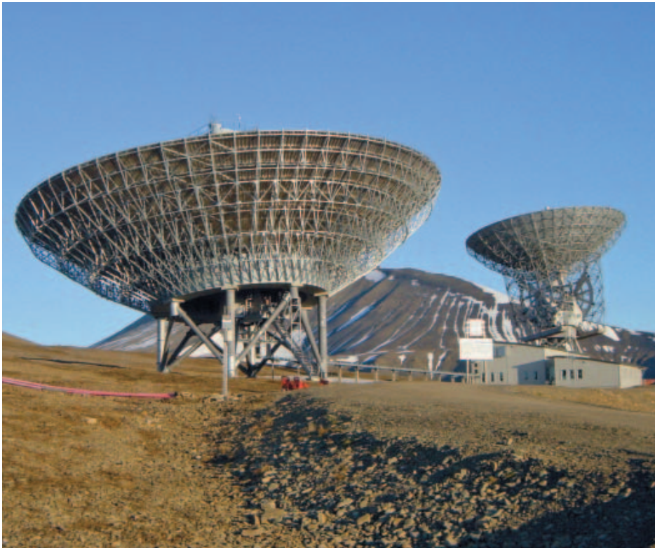
Figure 3. The two ESR (EISCAT Svalbard Radar) dishes on the island of Spitzbergen in the Svalbard archipelago. The one on the left is a 42-meter fixed dish and the one on the right is a fully-steerable 35-meter dish; each is capable of transmitting 500kW of coded pulses. These powerful radars are used by the APL team in conjunction with the UCL Fabry-Perot Interferometers on Svalbard and, particularly, the new SCANDI (Scanning Doppler Imager) instrument. (Image due to EISCAT).
