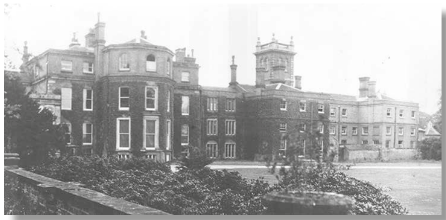
The Manor at Kings Bromley, home to the Newtons and later the Lane family, before it was pulled down in 1928.
