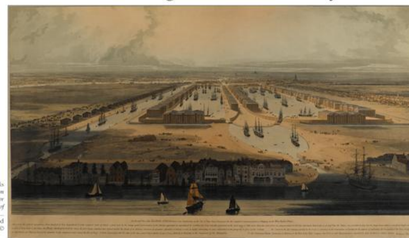
An Elevated View of The West India Docks & Warehouses near constructing on the side of Ships near Limehouse for the reception & accommodation of shipping in the West India Trade... Artist William Daniell, coloured aquatint and etching, 1802. © National Maritime Museum.
