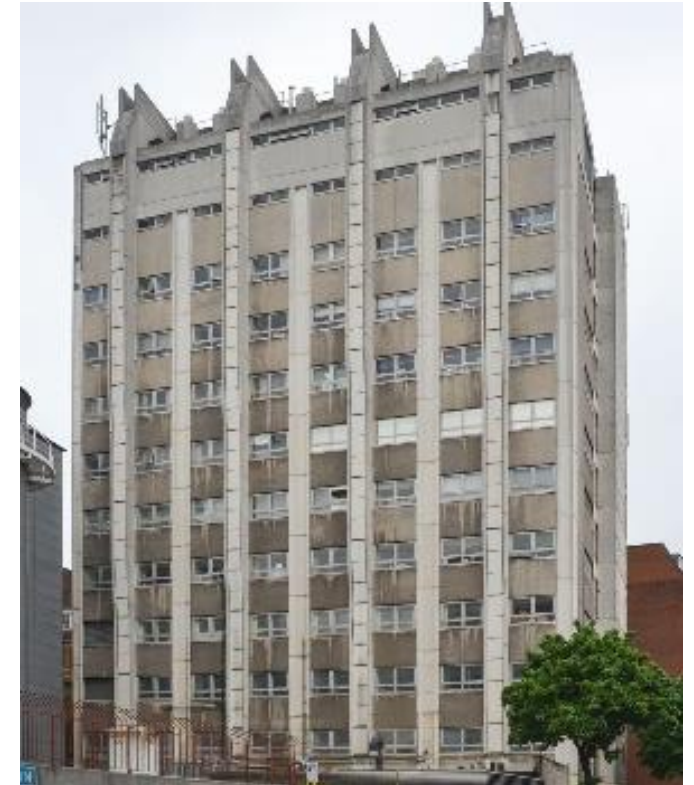
ION New Building! 1977
