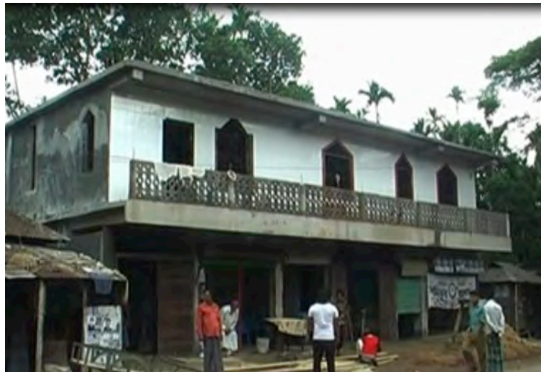
Figure 6: Construction of a Mosque in Sylhet, Bangladesh
