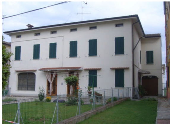
Figure 4.14 - Undamaged building adjacent to the building of Error! Reference source not found. in San Carlo.
