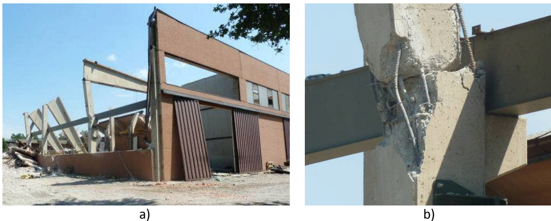
Figure 4.44 - Industrial buildings close to Mirabello: lateral panel failure.
