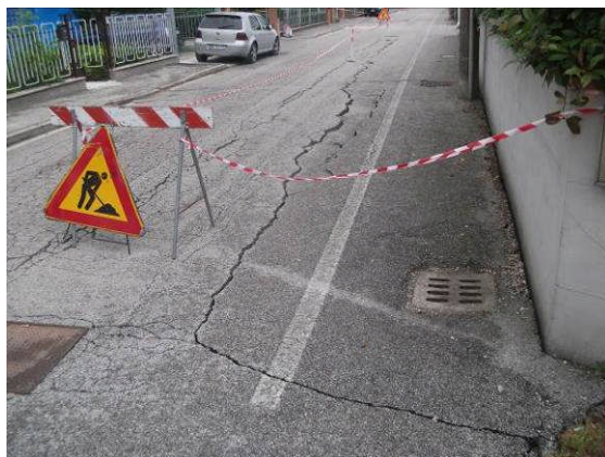
Figure 6.12 - a) Lateral spread and settlement in Via Argine Postale, Mirabello; b) lateral spread and settlement in Corso Italia, Mirabello; c) Surface cracks and damage to trench in Via Primo Maggio, San Carlo; d) Collapse of sub-base and subgrade, San Carlo.
