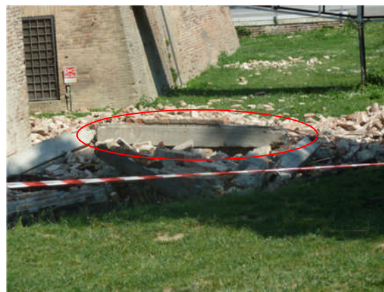
Figure 4.37 - Debris from the partial collapse of the tower of the Rocca Estense Castle.
