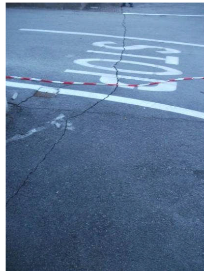
Figure 6.11 - a) Damage of house having access from 2 levels; b) Retaining wall adjacent to the house; c) detail of the damage of the pavement in front of the house.
