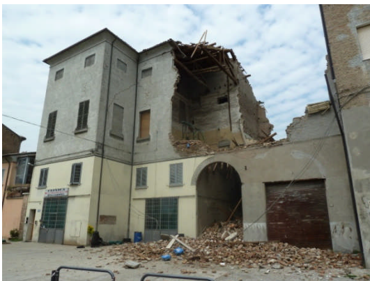
Figure 3.13 - Different degree of damage to residential building were observed in Finale Emilia. Damage was particularly evident for old and poorly maintained masonry structures.
