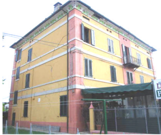
Figure 4.13 - Moderate damage of a commercial/residential building in San Carlo.
