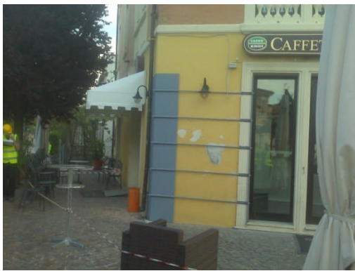
Figure 4.4 - Stabilisation of a commercial/residential building in Vigarano Mainardo.
