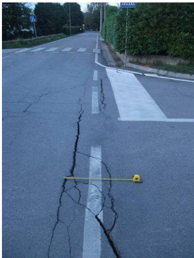
Figure 6.11 - a) Damage of house having access from 2 levels; b) Retaining wall adjacent to the house; c) detail of the damage of the pavement in front of the house.
