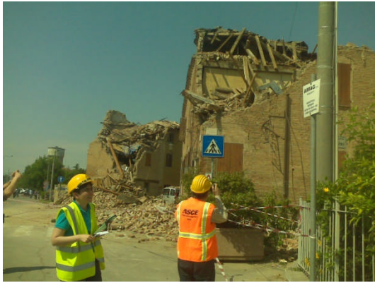
Figure 3.14 - Damage to historical buildings in San Felice sul Panaro. The ancient tower is collapsed and the castle presents fractures lines.
