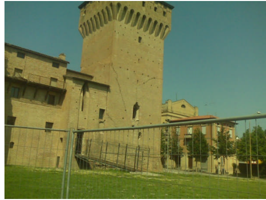
Figure 3.14 - Damage to historical buildings in San Felice sul Panaro. The ancient tower is collapsed and the castle presents fractures lines.
