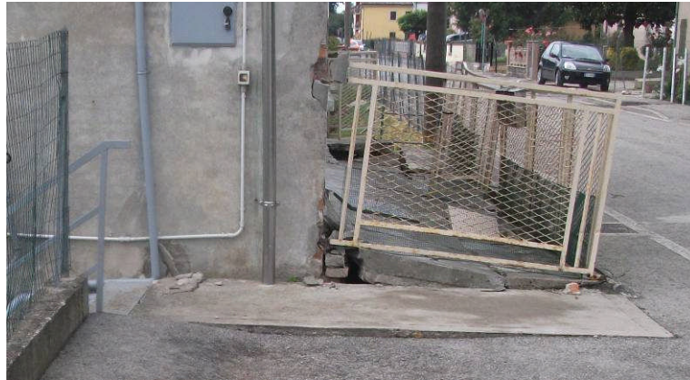
Figure 6.11 - a) Damage of house having access from 2 levels; b) Retaining wall adjacent to the house; c) detail of the damage of the pavement in front of the house.
