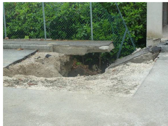
Figure 6.12 - a) Lateral spread and settlement in Via Argine Postale, Mirabello; b) lateral spread and settlement in Corso Italia, Mirabello; c) Surface cracks and damage to trench in Via Primo Maggio, San Carlo; d) Collapse of sub-base and subgrade, San Carlo.
