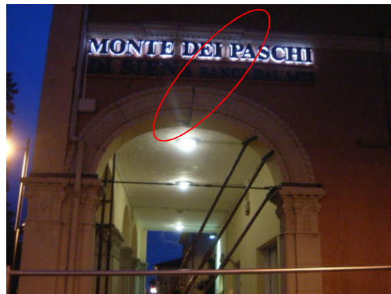
Figure 4.11 - Stabilisation to prevent overturning of the corner of a masonry building in Mirabello.
