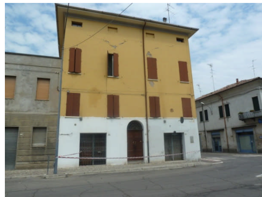
Figure 3.13 - Different degree of damage to residential building were observed in Finale Emilia. Damage was particularly evident for old and poorly maintained masonry structures.
