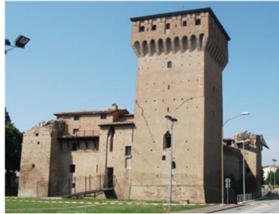
Figure 4.35 - Partial collapse of the two towers and severe damage in the third tower of the Rocca Estense Castle.
