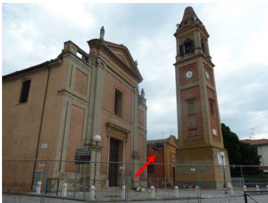
Figure 3.10 - Damage to the church of S. Agostino
