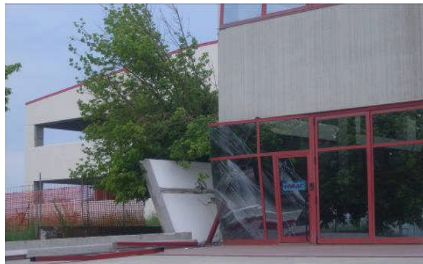
Figure 4.44 - Industrial buildings close to Mirabello: lateral panel failure.
