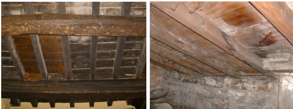
Figure 4.11: Timber floor and timber roofs.
