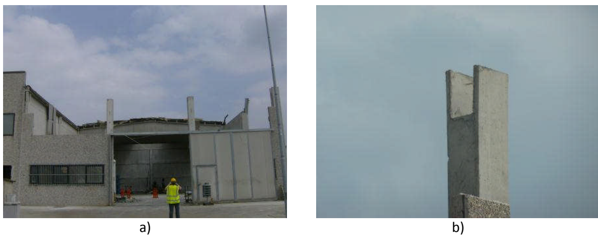
Figure 4.49 – a) Collapsed double T beam roof and prestressed concrete Beam of a warehouse at Casumaro b) Detail of a failed shear key connection.
