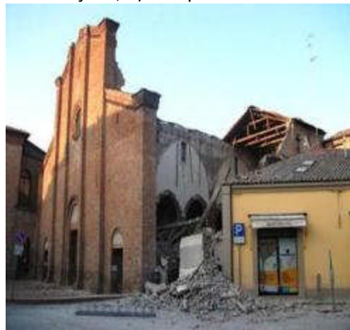
Figure 4.37 – Dislodged decorations from the façade and partial collapse of the roof and south side of the church of San Francesco in Mirandola.
