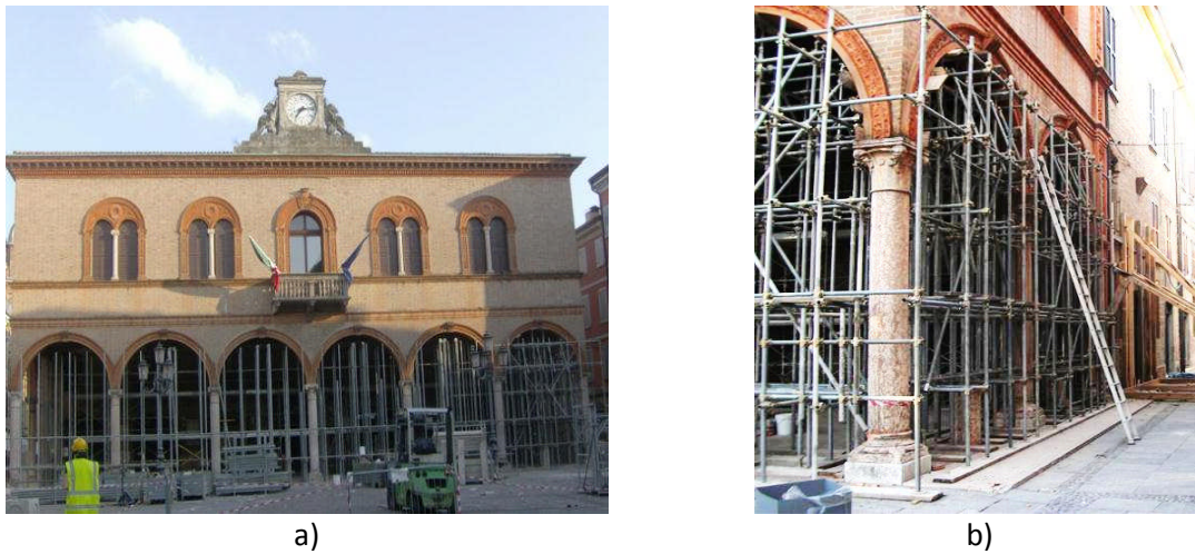
Figure 4.44 – Town hall in Mirandola: a) general view, b) side.
