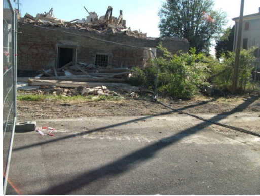
Figure 5.1 – Road closure due to fallen electricity cable.
