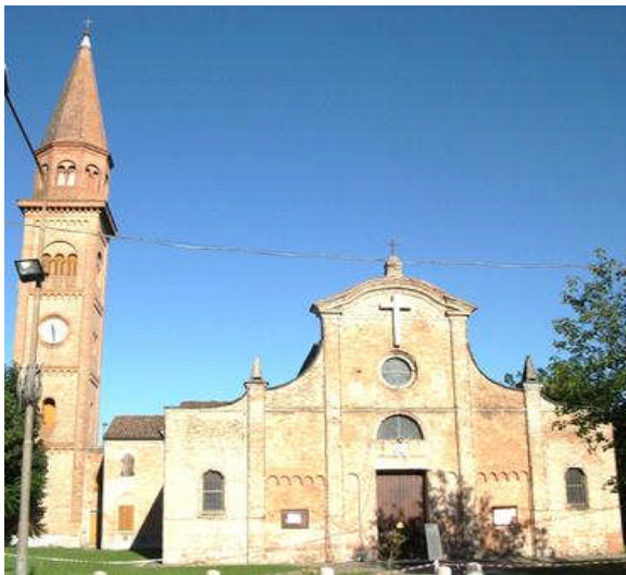
Figure 4.24 – Undamaged church of Pieve Matildica in Sorbara.
