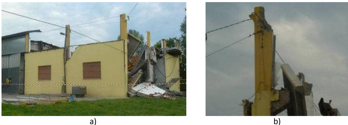
Figure 4.50 - Industrial buildings close to San Carlo: a) overview of the pre-cast structure; b) joint detail.
