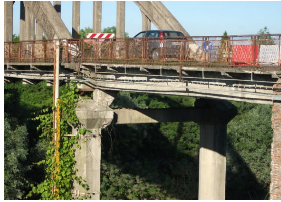
Figure 5.7 – Bomporto Bridge (reinforced concrete and masonry) open to traffic.
