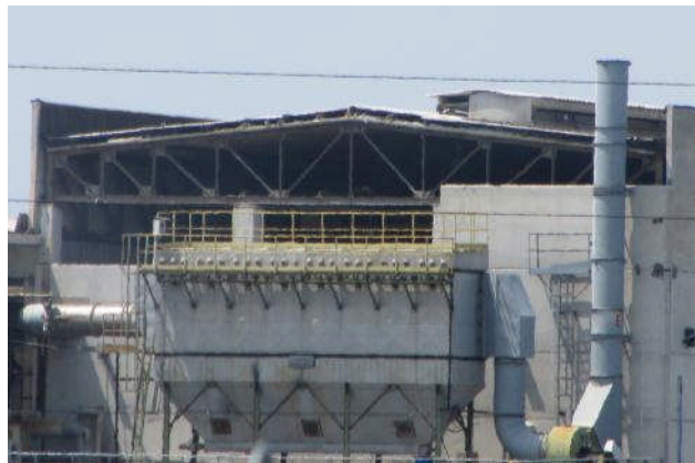
Figure 4.55 - Steel truss as the transverse support in a precast warehouse system close to San Felice sul Panaro.
