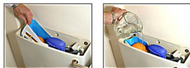
Installing water hippo
