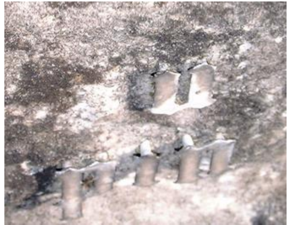
Figure 43 Lead lettering. Marble rock has been dissolved from beneath the letter to expose the pegs
