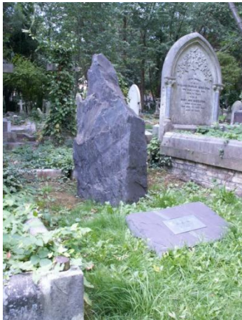
Figure 47 Slate memorial showing cleavage and original layering. (Highgate Cemetery)
