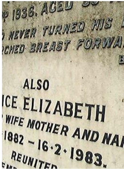
Fig 42 Lead lettering. The upper inscription is older, and therefore more raised, than the lower
