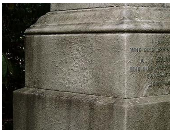
Figure 41 Weathered marble monument, showing discolouration, uneven surface and linear features. (City of London Cemetery)
