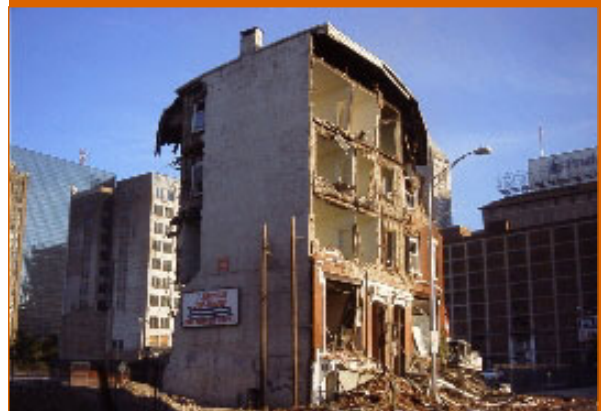
Photo: Demolition in preparation for the New Newark downtown development
