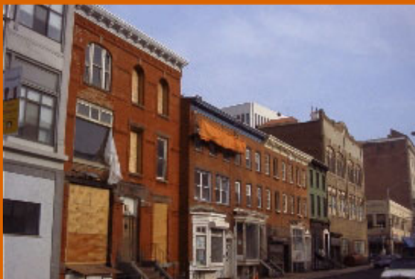
Photo: Renovations on Halsey St.
