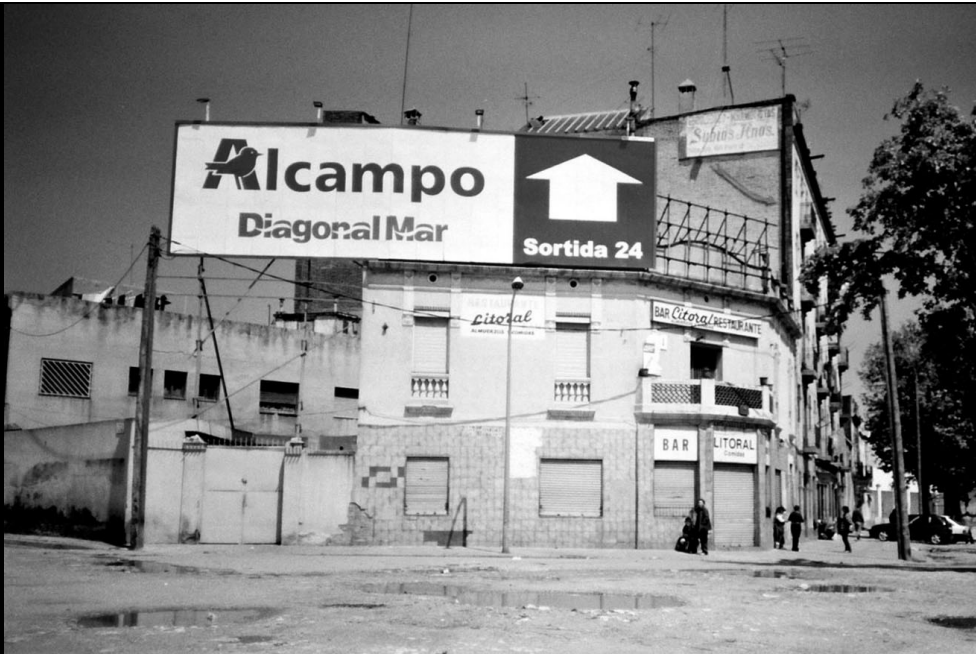
Photo 2. The Mina Housing Estate, in Sant Adrià del Besòs.
