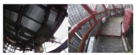
Fig. 17. Eddystone helideck views. Left: helipad, right: vertical structure rising from the gallery, with solar panels attached.
