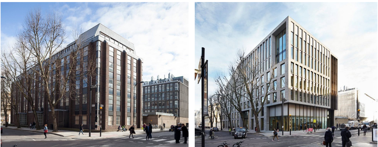
Figure 13 & Figure 14. Wates House before and after refurbishment. Photography credits: Matt Clayton and Jack Hobhouse
