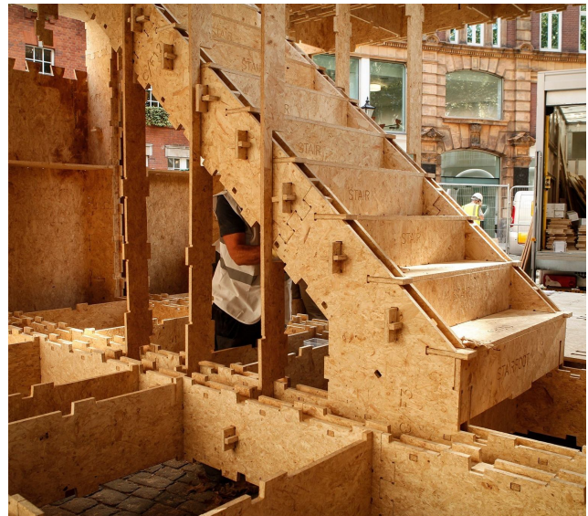
Figure 9 & Figure 10. Flat-packed CNC-cut timber components before and after assembly in the Wikihouse 4.0 prototype. Photography credit: Margaux Carron
