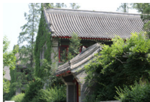
JINGYUAN 4, CLASSROOM BUILDING
