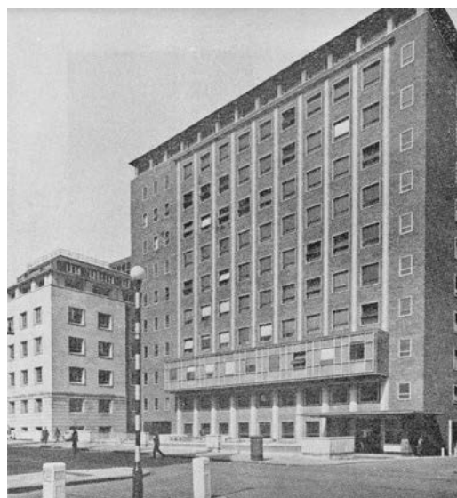
The "new" Engineering Faculty building (completed in 1961)
