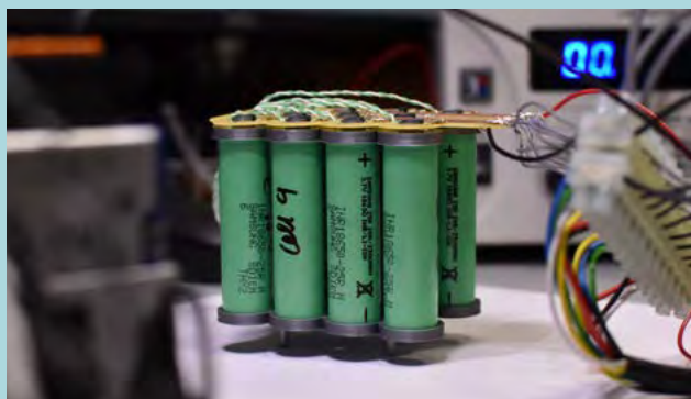
Lithium ion battery modules tested for hybridisation with other electrochemical technologies
