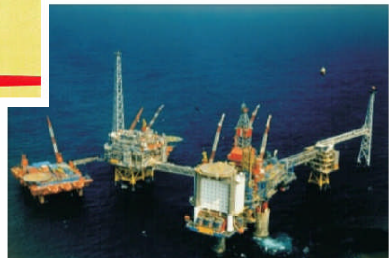
Sleipner West natural gas field where separated CO 2 is being injected into a deep salt-water reservoir (Courtesy of Statoil)
