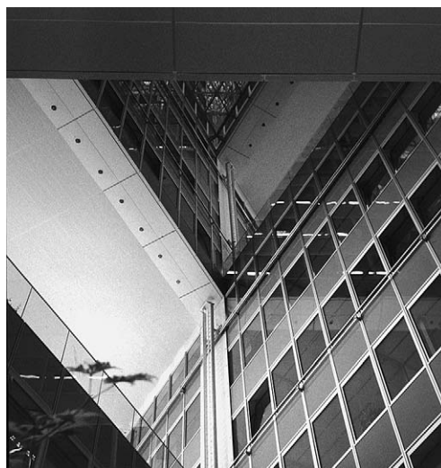
4. The Commerzbank atrium which provides daylight and natural ventilation to the building interior. (Courtesy of Steven A. Moore.)
