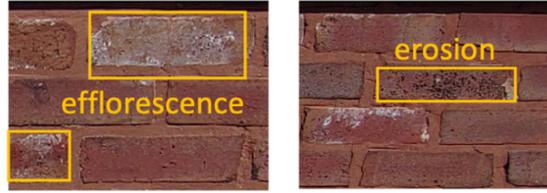
Figure 3: Images showing efflorescence and erosion defects
