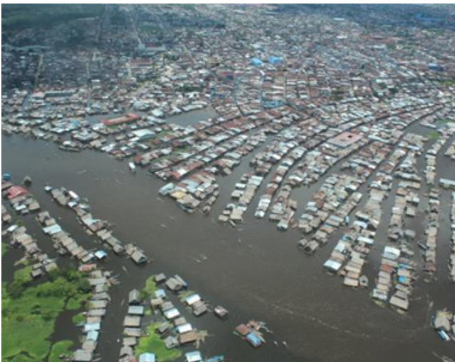
Flooding in the Lower Belen area
