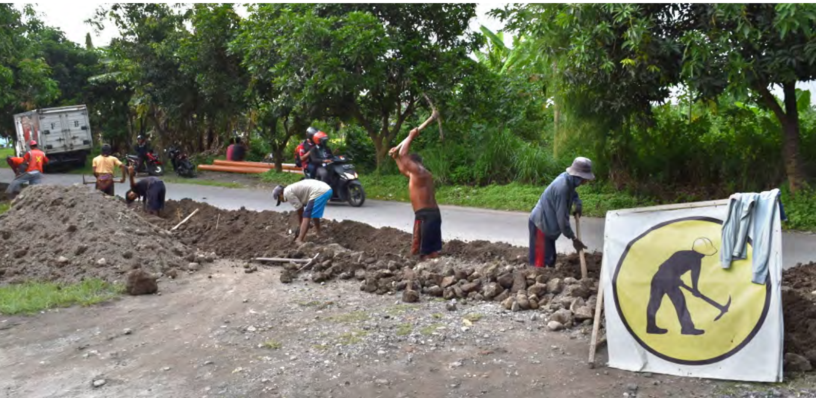
Picture 9. Sewerage works funded through Musrenbang, Solo, Indonesia Source: Kota Kita
