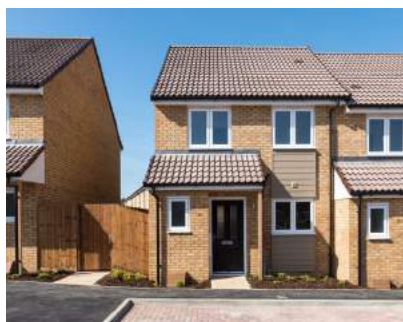
Paradigm's design & build site at Caleb Close in Luton. Caleb will deliver 224 affordable homes with a mix of rent, shared ownership and outright sale.
