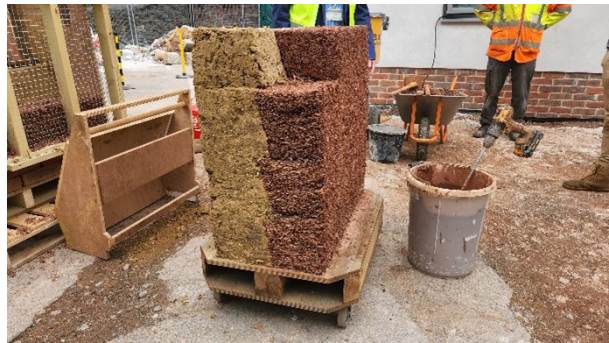
Section showing different cob mixes used in wall Image by Sadek Ahmed
