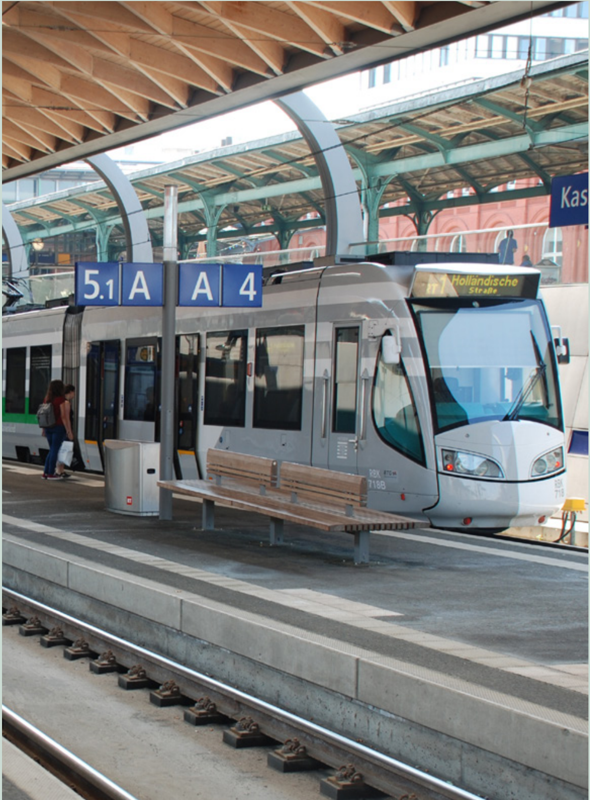
A new route has been developed under the Hauptbahnhof to allow the tram-trains into the city centre. Kassel, Germany
