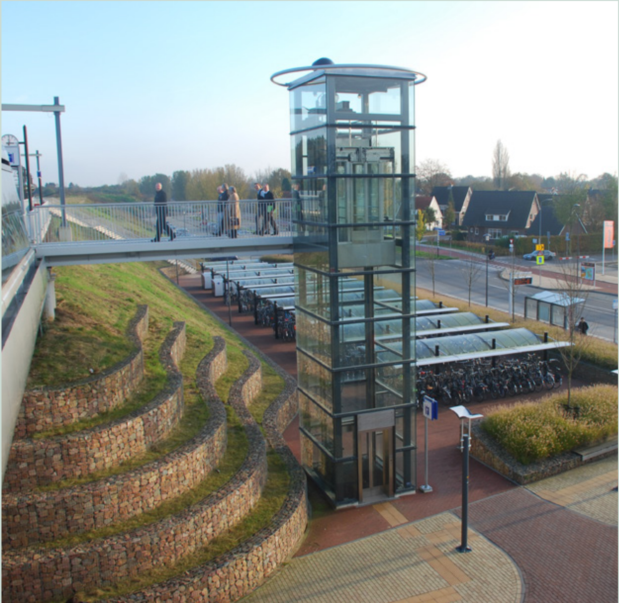
An exemplar small station improvement – a new station has been built to link the outlying village to Arnhem, leading to a revitalised local community. Westervoort, The Netherlands
