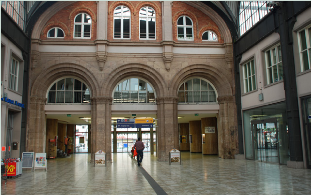
The refurbished Hauptbahnhof – now a cultural station with cinema, shops and restaurants. Kassel, Germany
