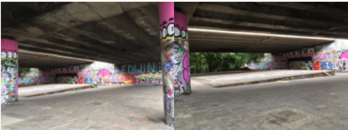
The disused motorway undercroft of the A12 flyover.
