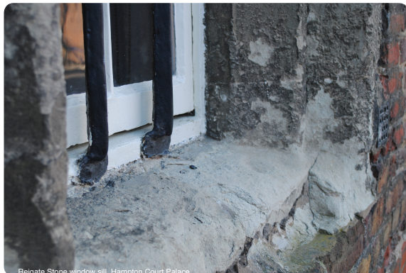
Reigate Stone window sill, Hampton Court Palace
