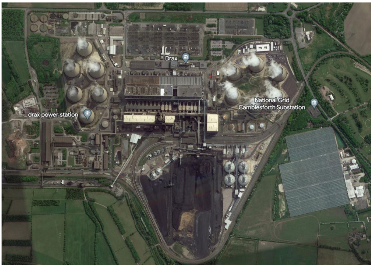
Figure 22 : Drax power station
