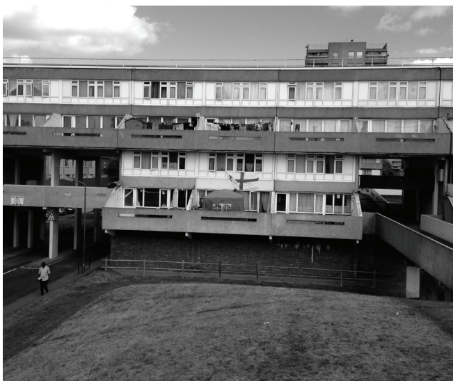
Figure 4.3. Buildings in Thamesmead elevated to first floor level approached via raised pedestrian bridges. Source: Author (2016).
