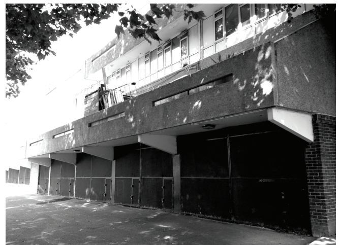
Figure 4.10. Garages at street level Source: Author (2016).
