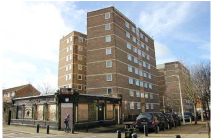
Figure 16. Abandoned pub in North Woolwich
