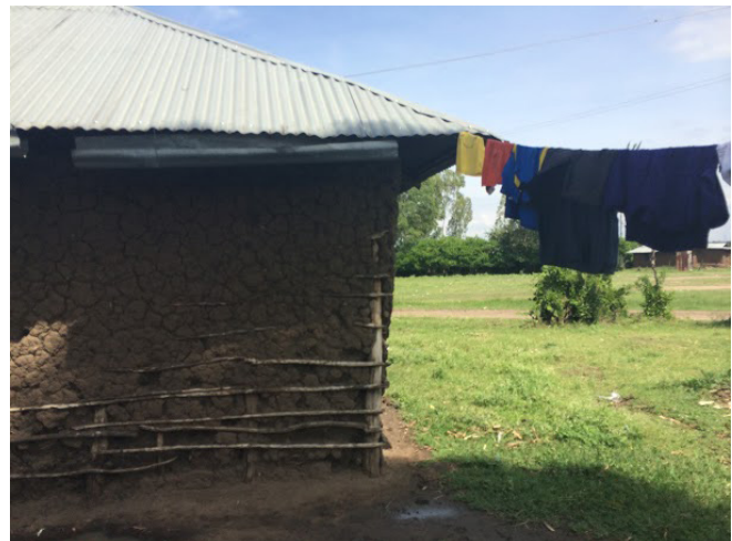
Picture 2. Mud and wood housing, Dago Unit, Nyalenda. Photo credit: Kai Mao.
