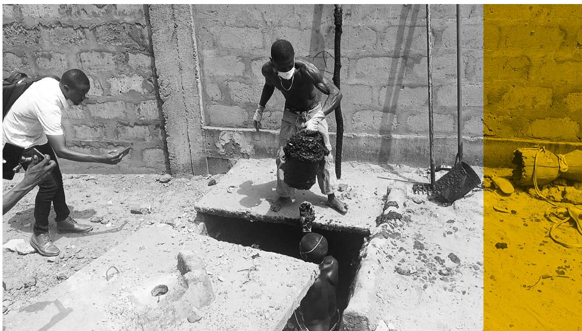
COMMIT: Realising the right to sanitation requires recognition of the makers of sanitation. Here a manual pit emptier services a household in Freetown. Photo Credit: OVERDUE 2021.
