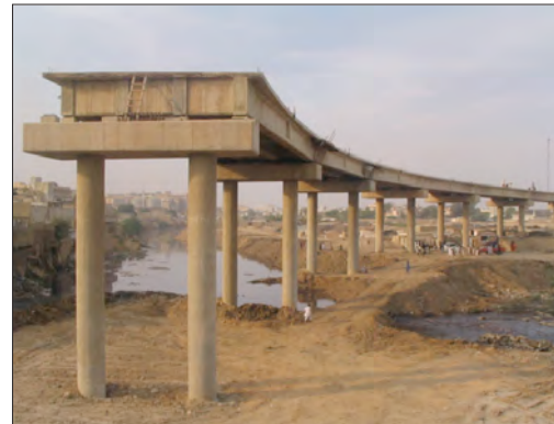
Picture 4: The construction of the LEW is underway.
