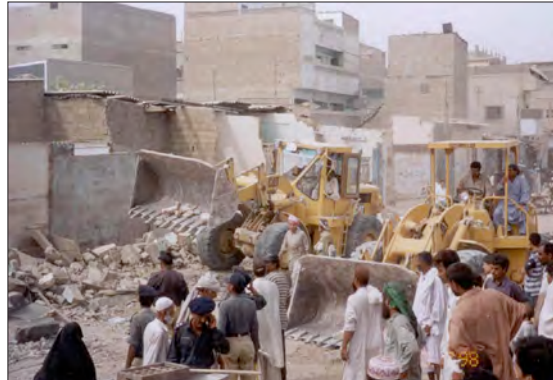
Picture 3: The demolitions.
