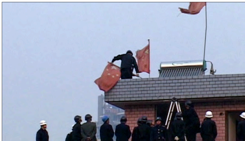
Picture 8: the Police removing flags the residents hoisted on the roof of their home before proceeding with demolition. This image is captured from a video film taken by one of the residents.
