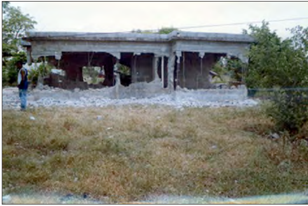
Picture 1: 2004. Demolition of a home in el Barrio Valiente.
