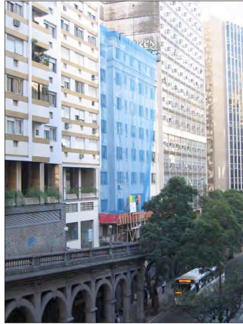
Picture 6: 14 July 2008, the building is being renovated.
