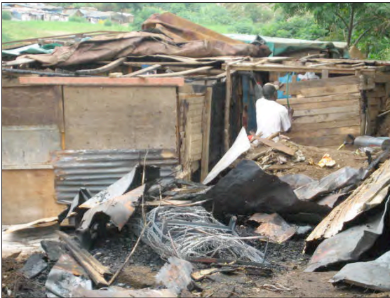
Picture 3: January 2007, rebuilding after a shack fire in Kennedy Road.
