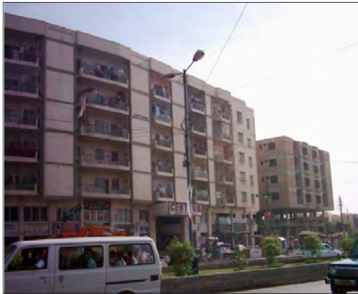
Picture 5: Views of one of the resettlement sites. Source: Urban Research & Design Cell at the Department of Architecture and Planning, NED University of Engineering and Technology, Karachi
