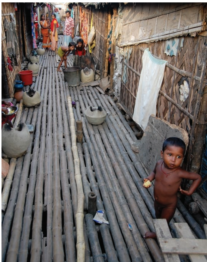
Left: Rental rooms in Mohammadpur, Dhaka are built-up over the water and the central walkways are made of bamboo (Huraera Jabeen, 2009)
