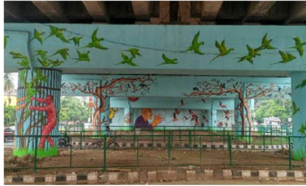
After intervention Figure 22: Example of flyover, India
