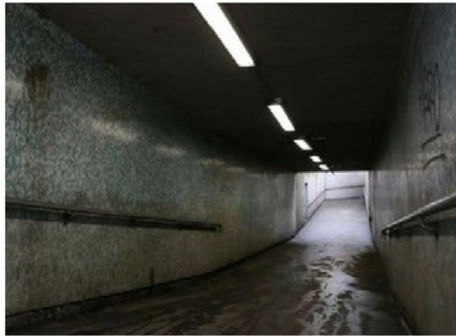
Before intervention Figure 18: Intervention- underpass: present
