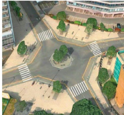
After intervention Figure 10: Intervention- intersection 1
