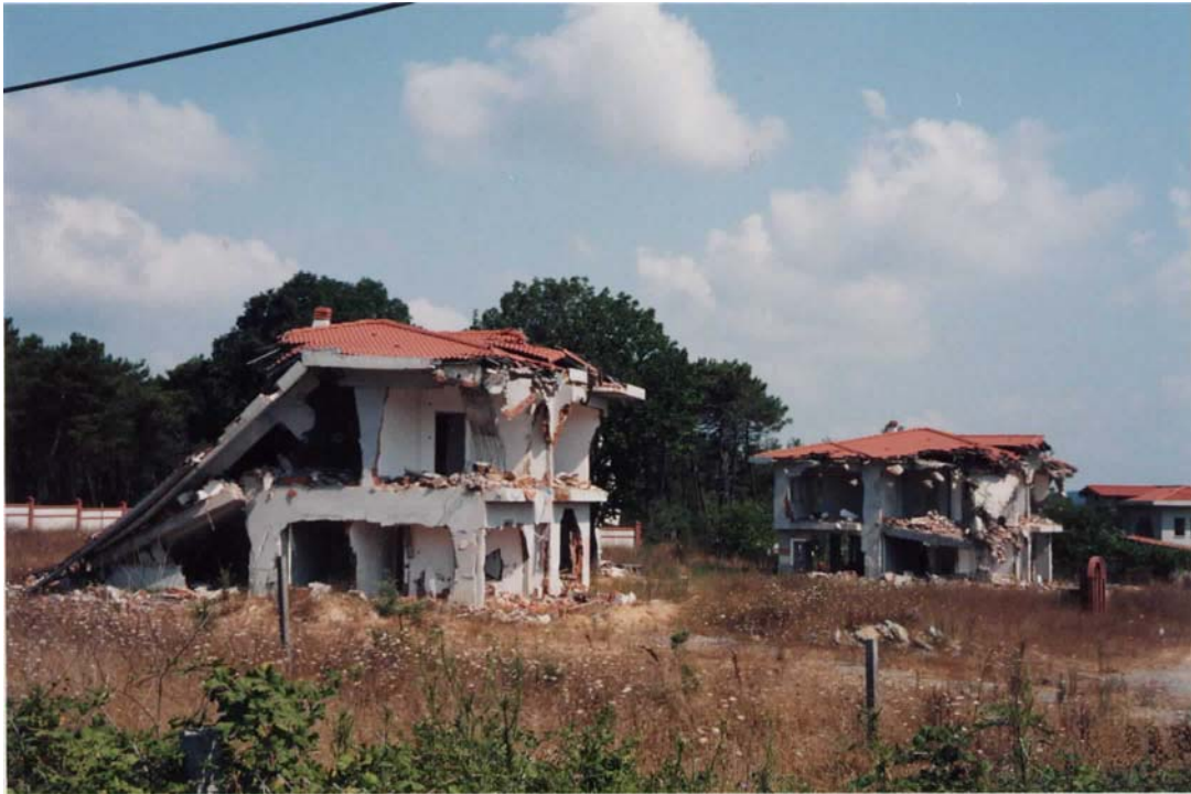
Plate 3: Buildings within Ömerli watershed demolished by ISKI (29/07/01)
