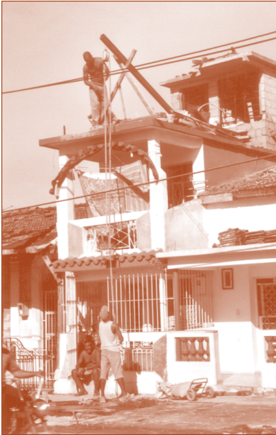
People repairing and expanding their houses in the Barrio Pogolotti, Havana
