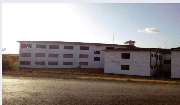
Bong Community College under construction
