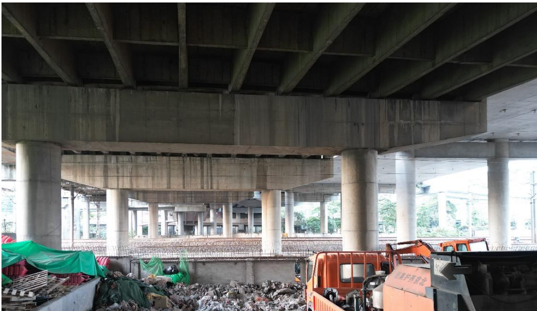
Figure 3: Complex under-bridge environment
