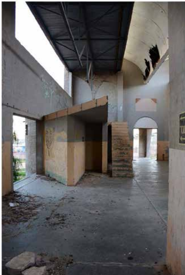
Figure 2: Steinkopf Community Centre interior
