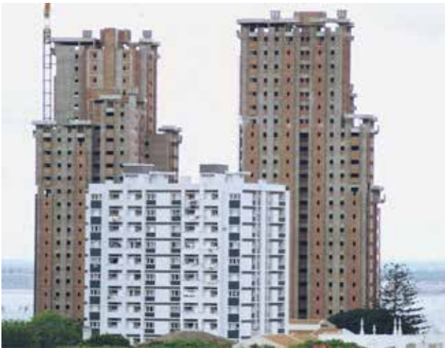
Figure 3: The construction of the Torres Vermelhas left unfinished after Independence ( http://kundalini-pt.blogspot.com/2007/04/maputo-ontem-lourenomarques.html ).
