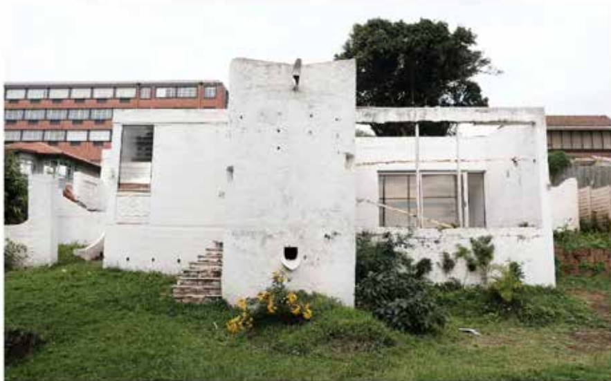
Figure 5: House Biermann, showing the state of the West facade (Silvia Bodei, 2021)
