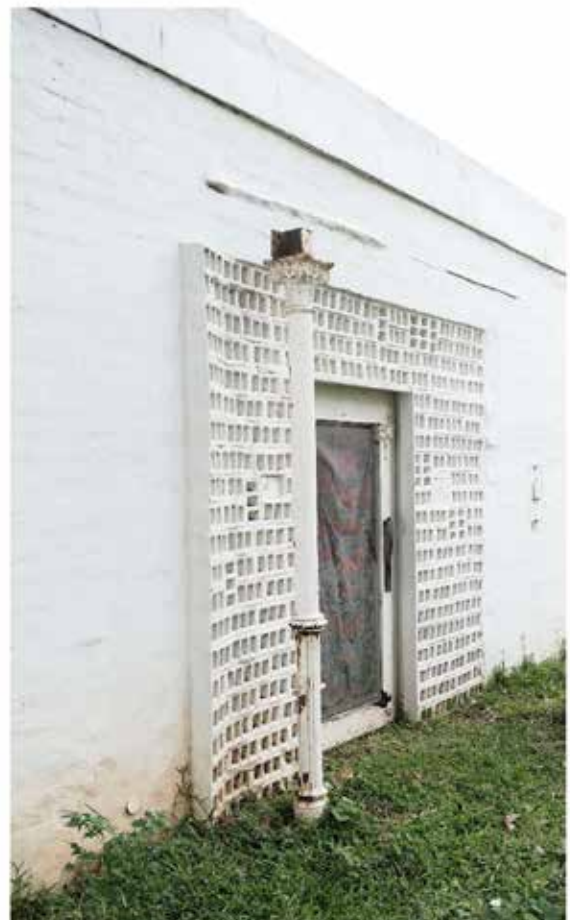
Figure 4: House Biermann, picture of the current state of the entrance with the detail of the Corocell bricks placed on edge and reversed. (Silvia Bodei, 2021).
