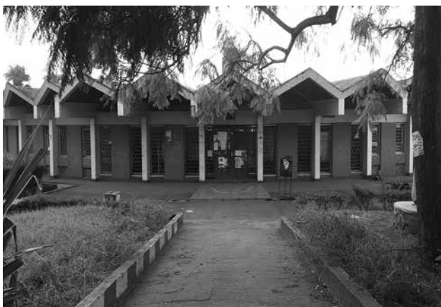
Figure 4: Kyambogo University (originally Uganda Technical College), Kampala, Uganda (1958), Photo: Year and photographer unknown.
