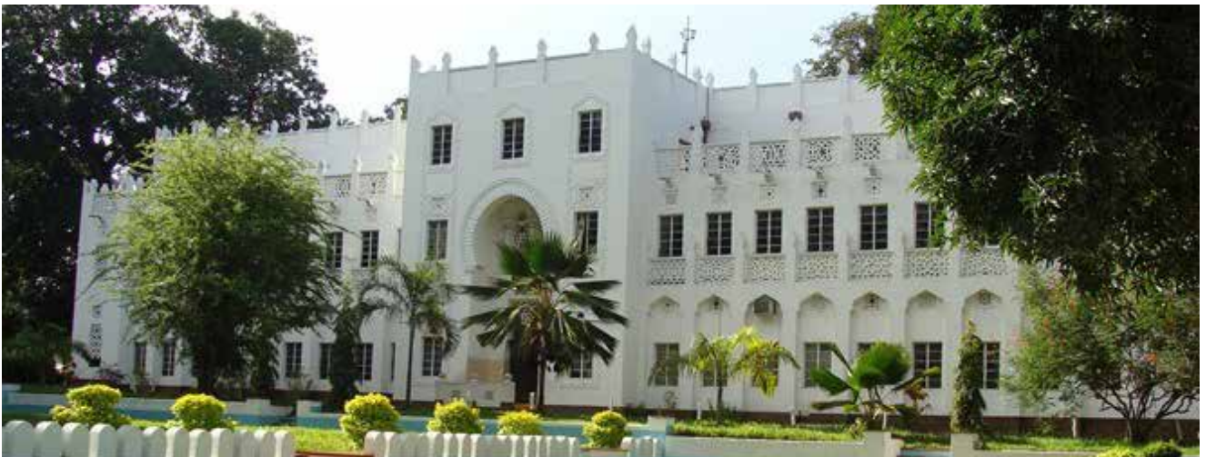
Figure 5: Pwani University building (source, Okoko).
