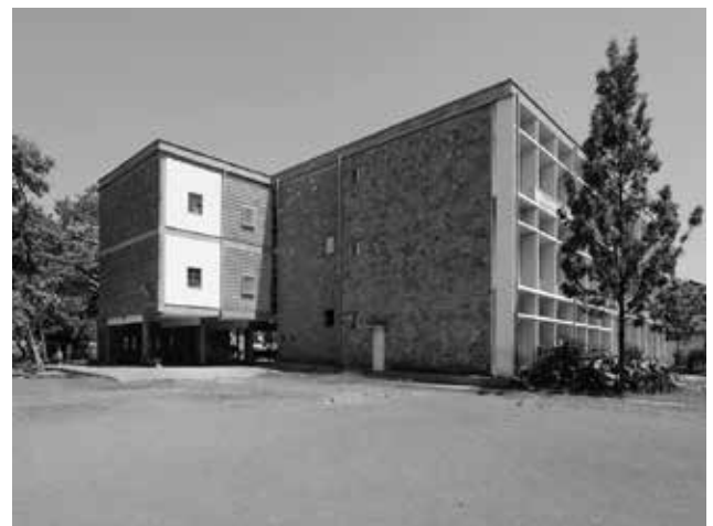
Figure 3: Girls' School Aga Khan (Mädchenschule), Kisumu, Kenya (1949-51), Architect: Ernst May, Photo: 2018 © Jean Molitor.
