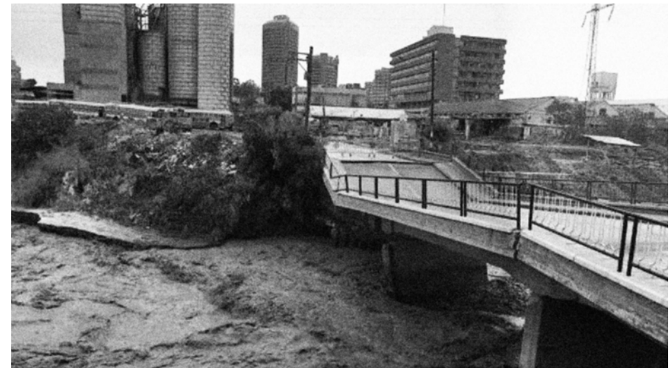
Collapsed bridge, Flood of the Ayalon River, 1954
