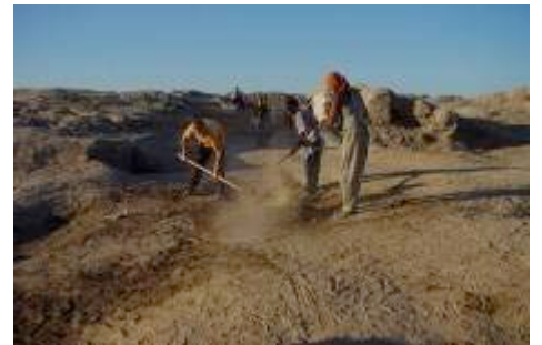
Preparing the material for backfilling.
