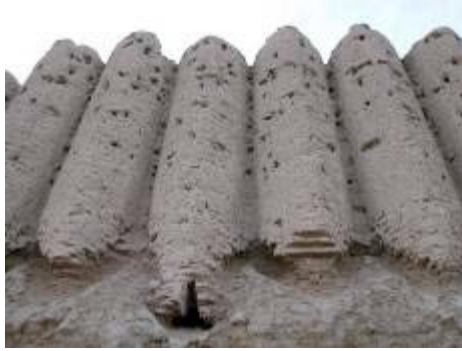
Great Kyz Kala. The 'corrugated' walls of the köshks make the walls more difficult to attack, allow rainwater to run off them without damaging the walls and help protect the inside from heat in the summer and cold in the winter.
