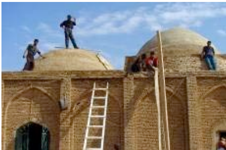
Replacing earlier conservation work on the roof of Ibn Zayd.
