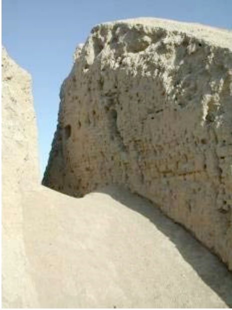
A cut through the defensive wall at Erk Kala shows its construction of carefully-laid mud bricks.
