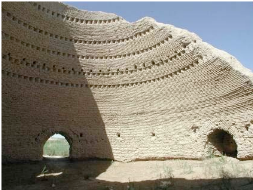
Decorative patterns inside the mudbrick dome of an icehouse in Merv. The two entrances you can see are where ice and snow was taken in for storage.
