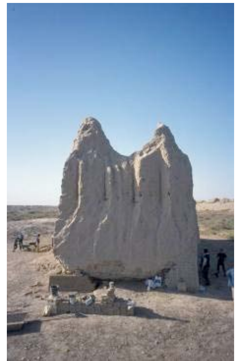
Restoration work at the Kepter Khana in Merv.
