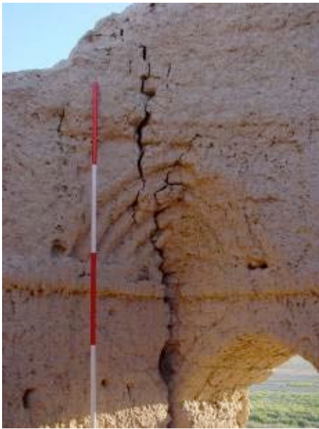
Little Kyz Kala. This cone-shaped feature was specially designed to connect the upright walls of this room to a domed roof. Each section of the rod measures 20cm.
