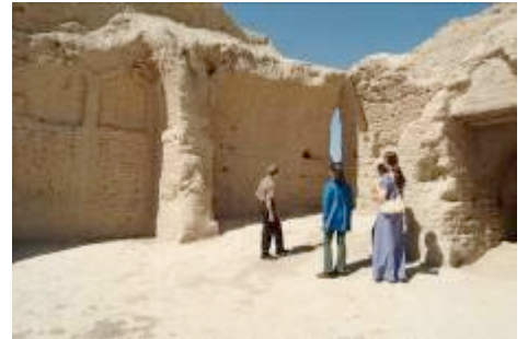
Vaulting in the walls of the Great Kyz Kala is evidence for domed roofs. Decorative brickwork can be seen on the left of the photograph.
