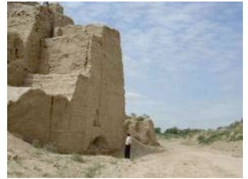
This photograph, taken from inside the walls, clearly shows the gallery walkways which allowed soldiers to patrol and defend Gyaur Kala at different periods.
