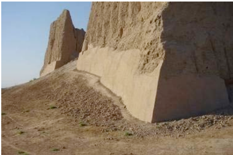
An eroded wall base at the Great Kyz Kala repaired with new mudbricks and replastered.
