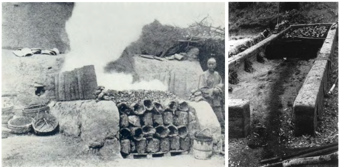
Figure 8.1 Left: a crucible iron smelting furnace in operation in Gaoping county, Shanxi province (Wagner 2008, 40); right: a rectangular furnace for crucible iron smelting, partly loaded with crucibles packed in coal in Hunan province (Wagner 1995, 151).
