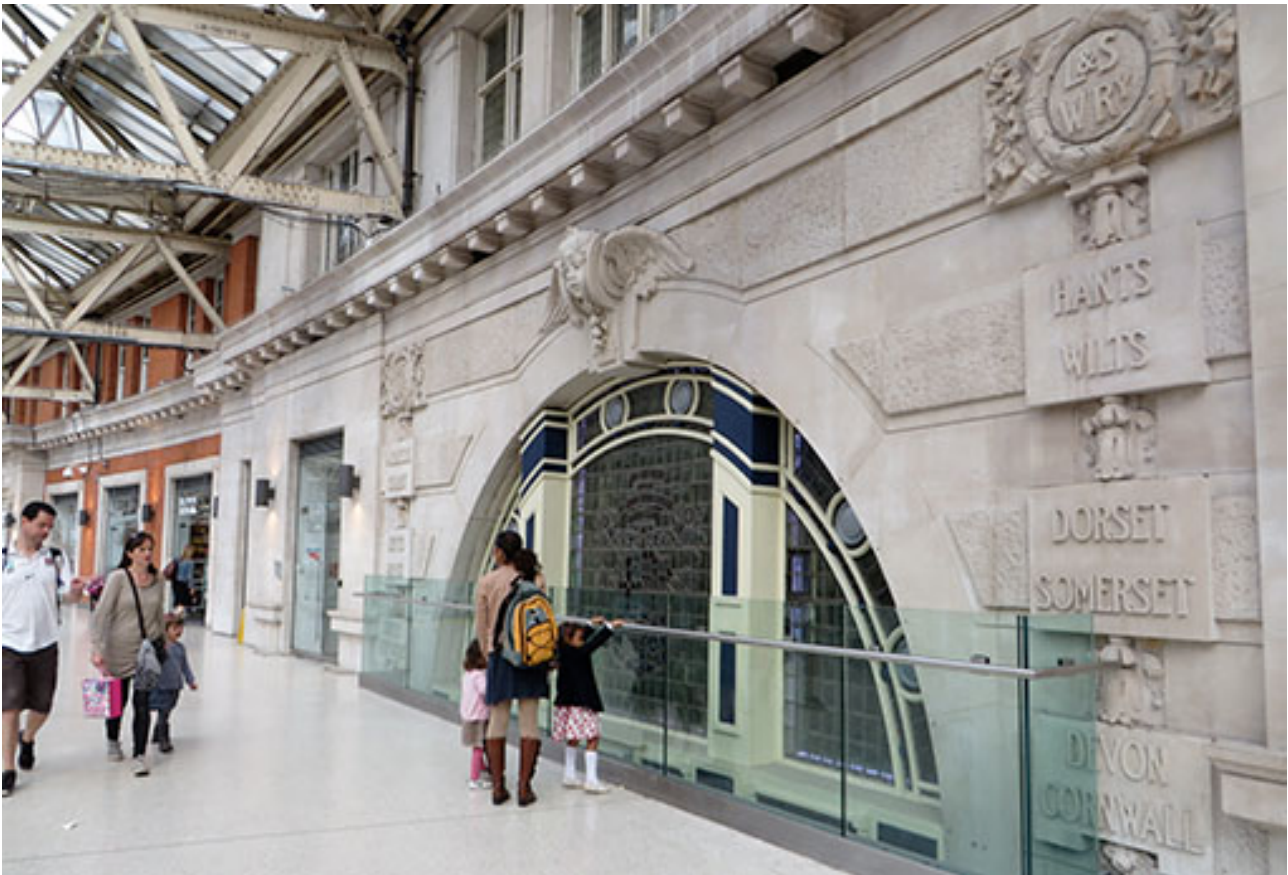
Waterloo Station: Portland Whitbed on the balcony level.
