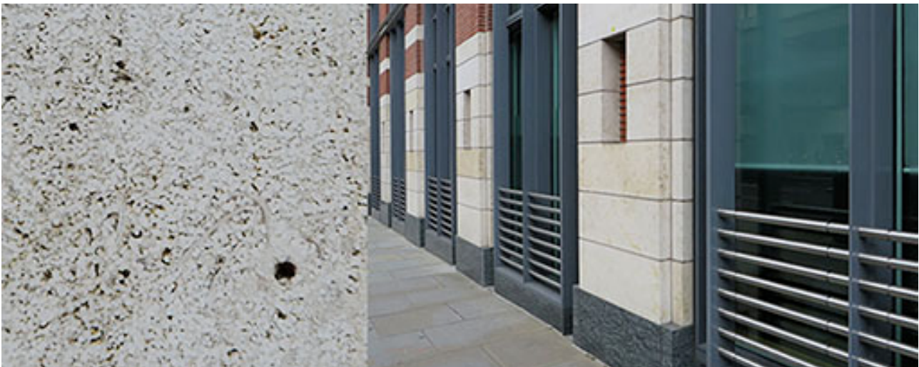
Left: oolitic limestone on the façade of 160, Queen Victoria Street (right). The dark green Verde Maritaca is seen in the foundations.
