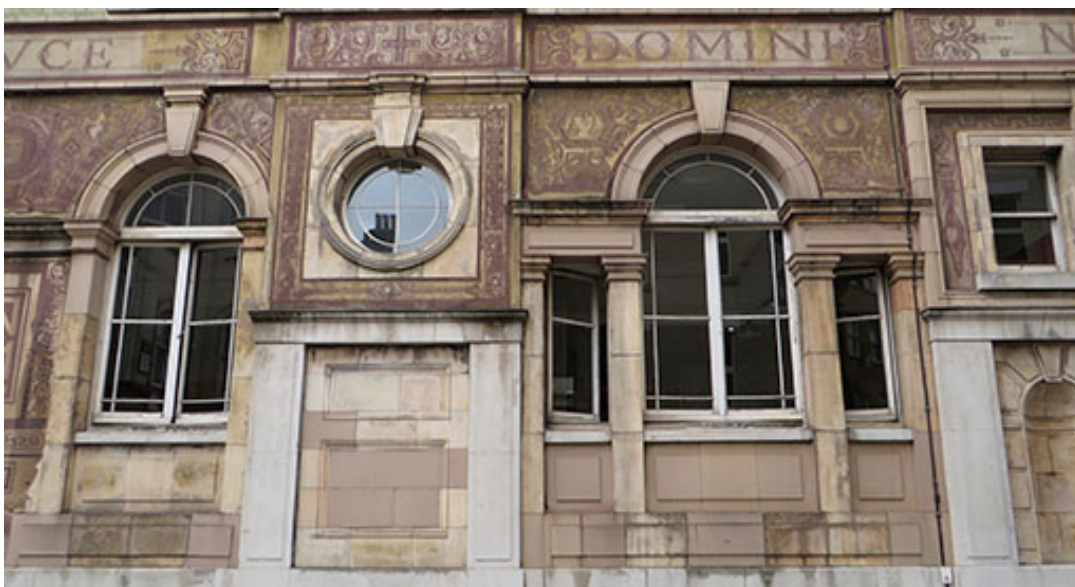
Carter Lane YHA, formerly St Paul's Choir School. Note the masonry using red sandstone below the windows.
