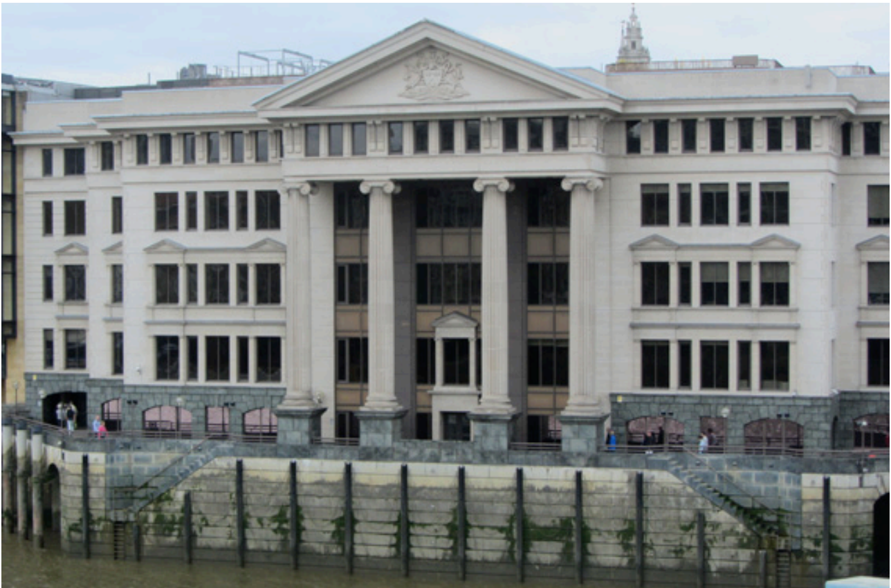
Vintner's Place, rear elevation facing the Thames.
