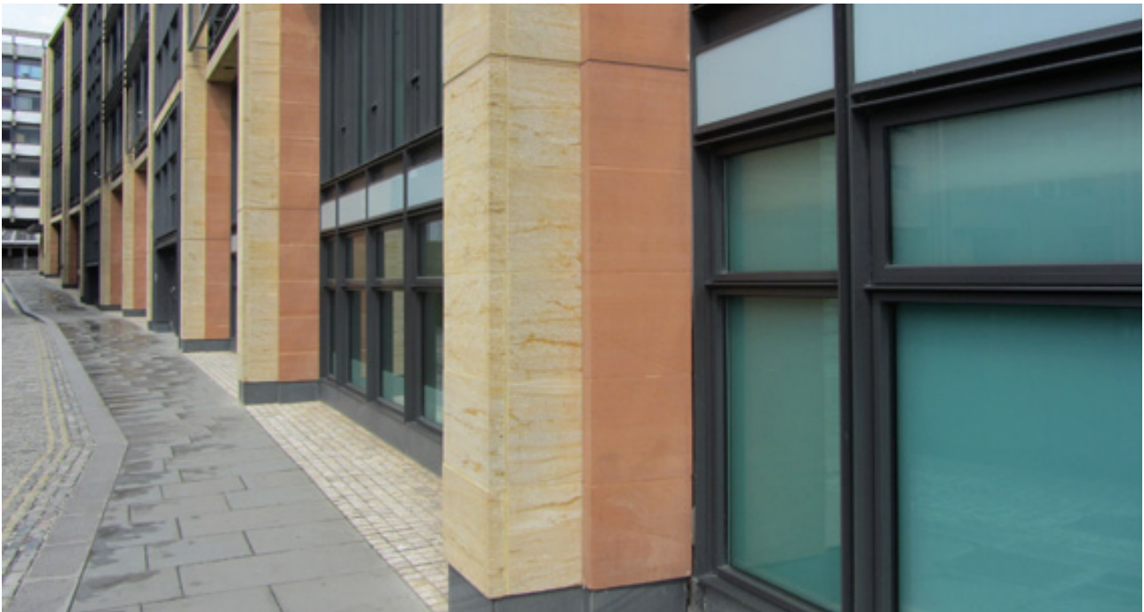
Thames Court, Queenhithe: red Corsehill Stone and yellow Ham Hill Stone clad the pillars on the exterior.
