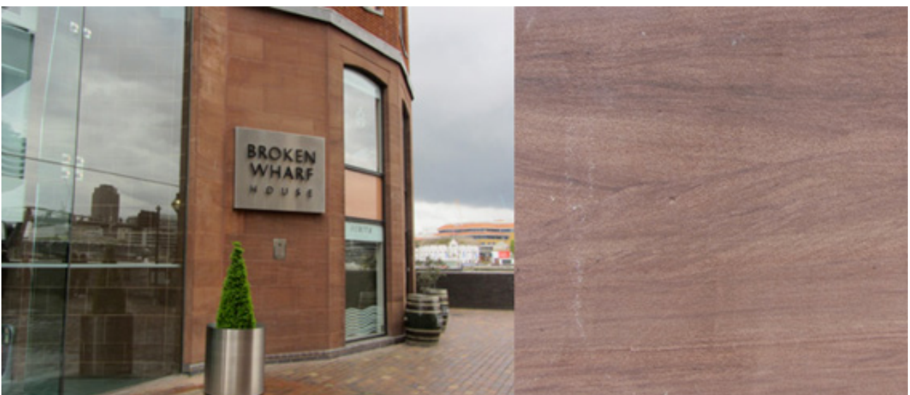
Left: Broken wharf House; Right: Channel cross bedding in the sandstone (upside down!).
