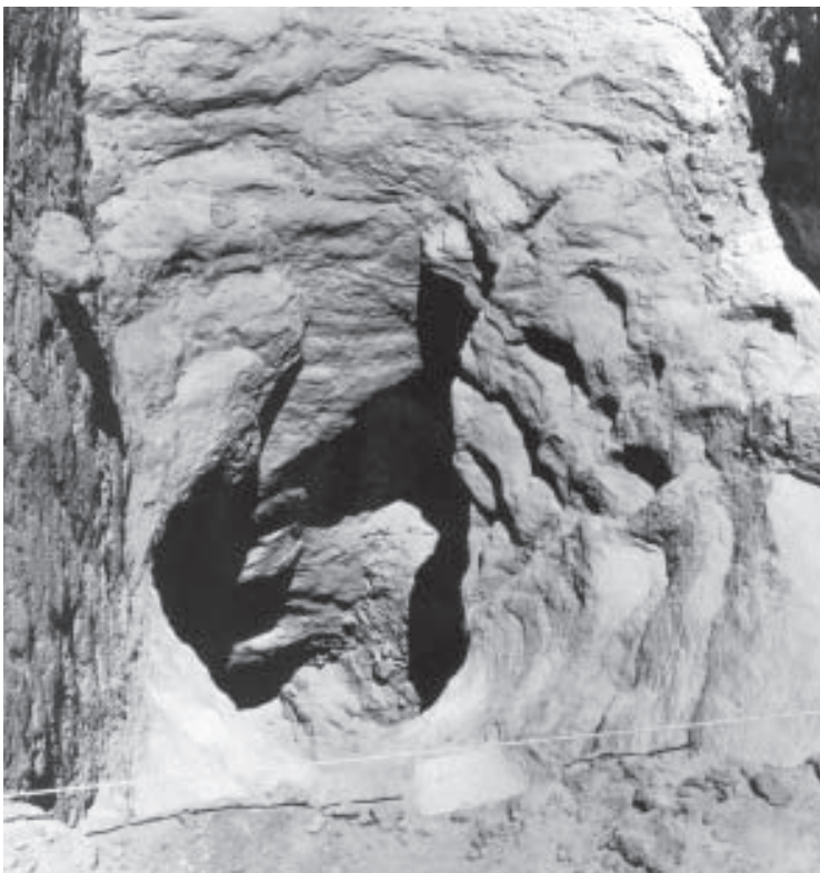
Fig. 8. Shaft T32 - typical for shafts used for the movement of miners and ores.
