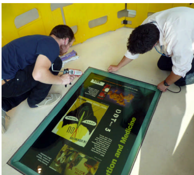
Adam polishes the glass while Daniel removes the lifting tapes and rings.
